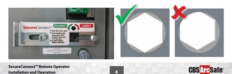
4. Rotate the knurled locking knob on the right side of the Remote Operator until it clicks and stops rotating, and then depress the ¼" tool head on Remote Operator until it locks in place. This will facilitate easier installation of the Remote Operator.
